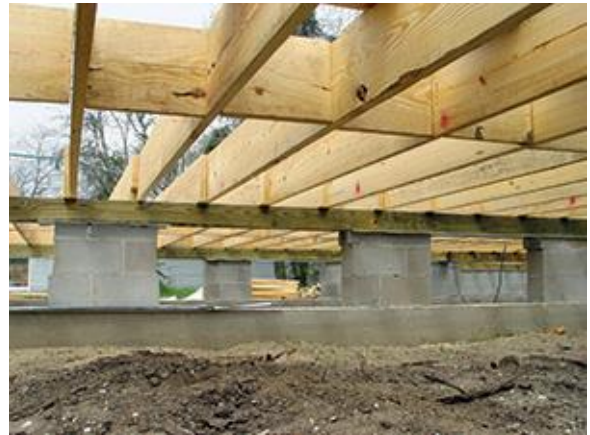
Figure 11: Pier and Beam Foundation
